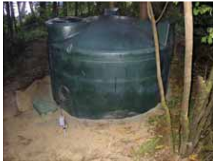
Tank with valve box (on left) backfilled with 10-inch fill.
