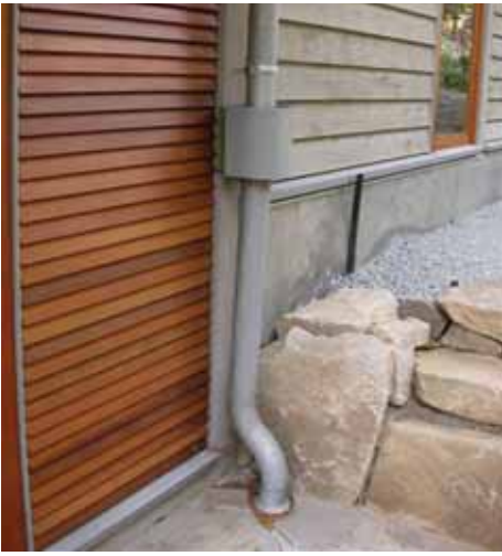
Debris pail above standpipe to underground transport piping. Low steel debris pail.
