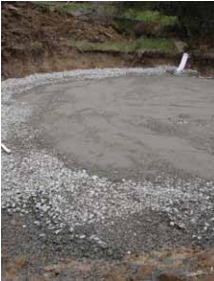
Compacted tank pad for steel cistern.
