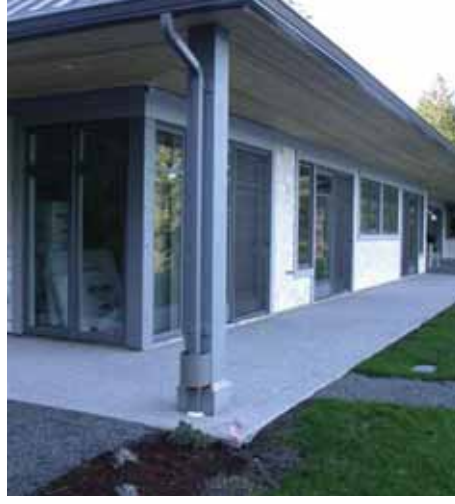
Debris pail above standpipe to underground transport piping. Low steel debris pail.
