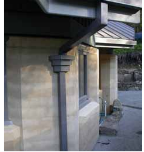
Custom-designed debris catchment box.
