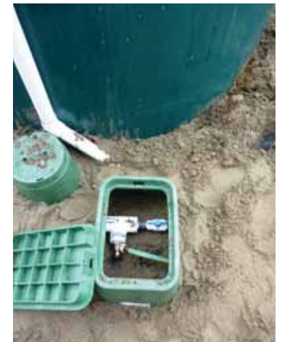
Partially backfilled valve boxes.
