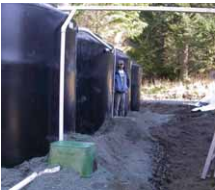
Four poly 11,365 L (2500 gal) tanks, partly backfilled.
