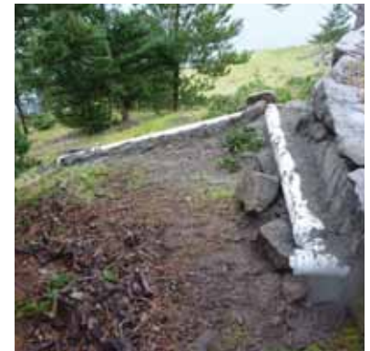
Large, underground FFD pipe partly backfilled.
