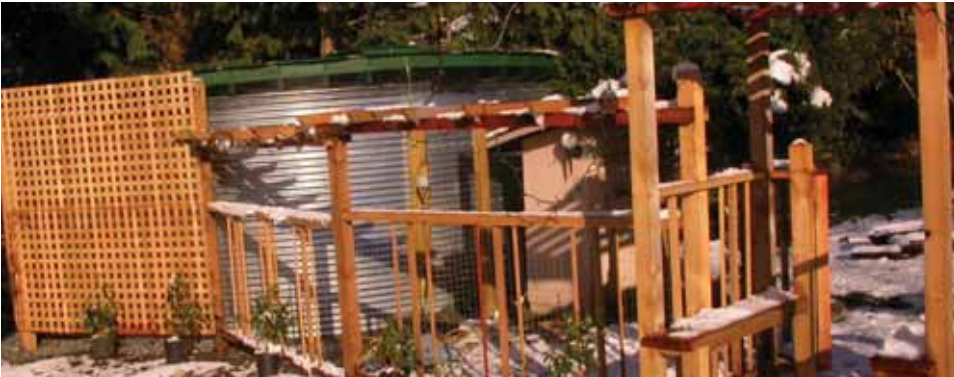
72,700 L (16,000 gal) steel tank behind trellis.
