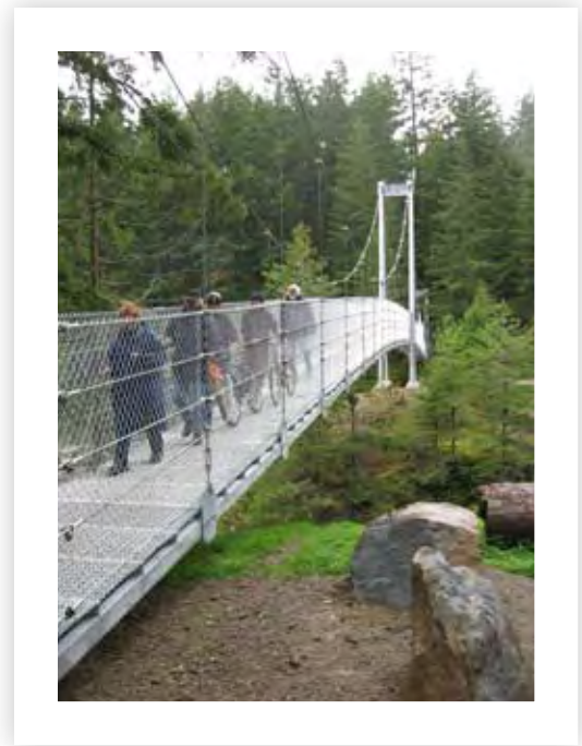
Top Bridge Crossing, cable suspension bridge, Englishman River Regional Park.
