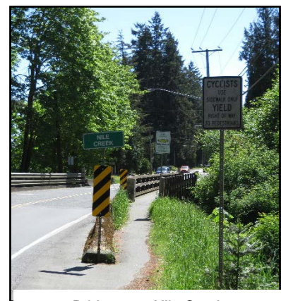
Bridge over Nile Creek
