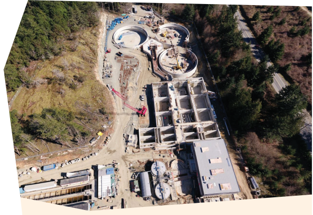
Secondary Treatment Upgrade at Greater Nanaimo Pollution Control Centre
