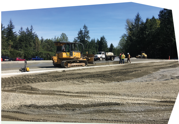
Mount Benson Regional Park new parking lot construction project
