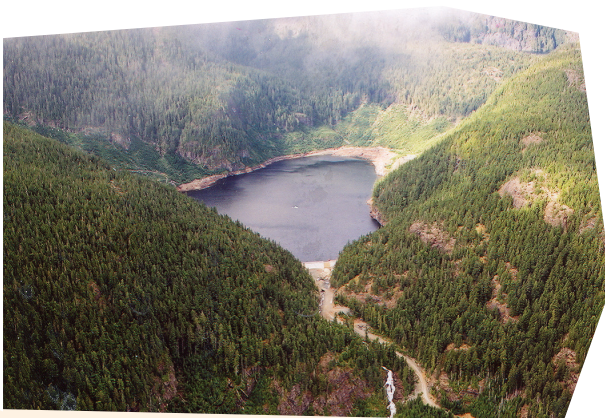
Arrowsmith Water Service Reservoir
