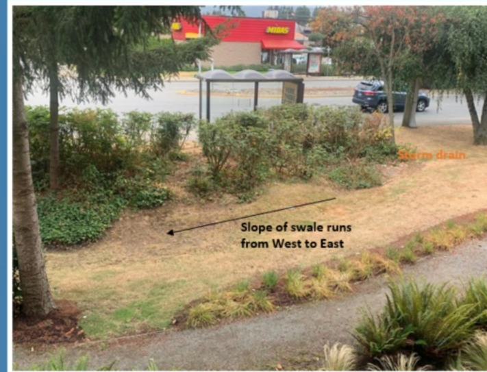
RDN Rain Garden – overlooking the West side of swale from RDN Admin Building
