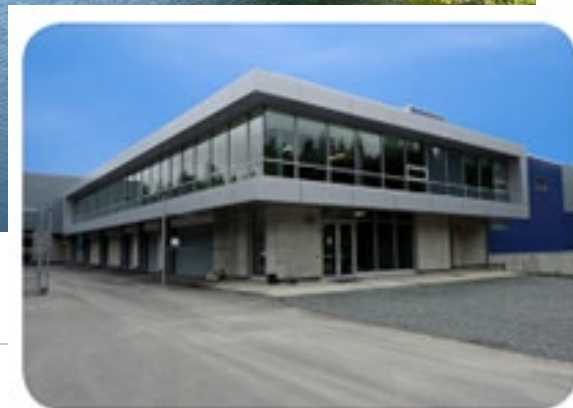
CoN Water Treatment Plant
