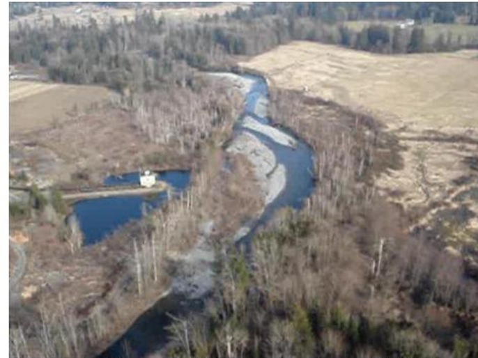
3.) Airphoto of Harmac Well looking downstream at 2+300m.
