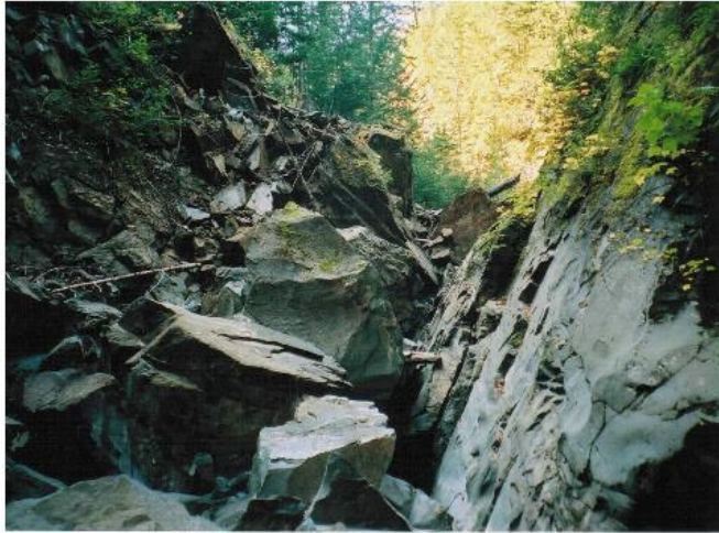
5.) Large debris slide plugging creek looking upstream at 16+976m.
