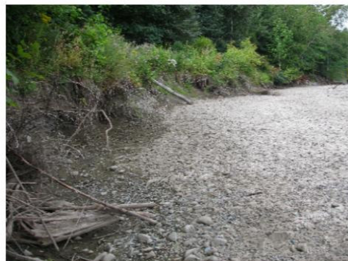
4.) Right bank erosion site looking upstream at 2+400m (2009).
