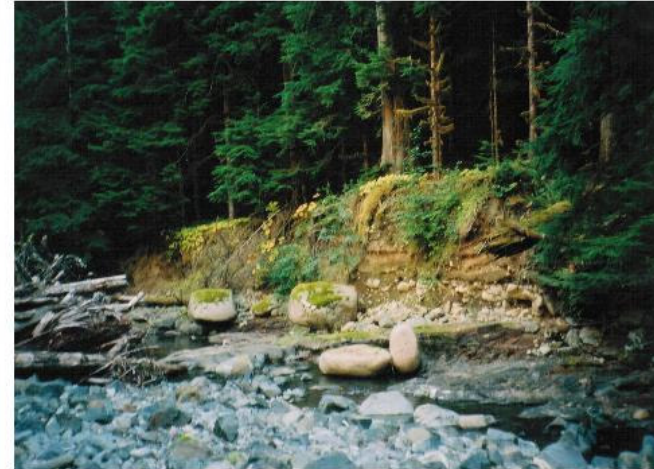
3.) Left bank erosion site at 15+835m.
