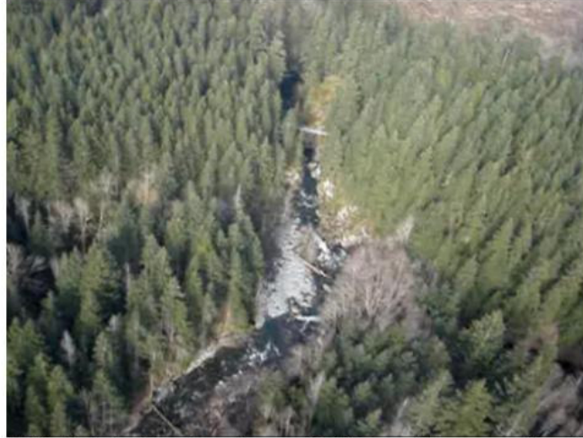
1.) Airphoto looking downstream at 8+100m and lower reach break.
