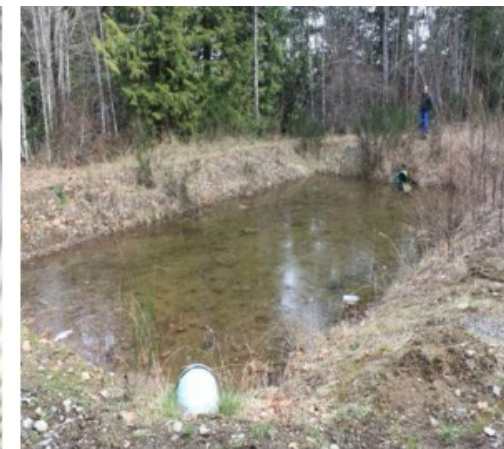
SHELLY CREEK: Baffled culvert and sediment retention pond installed under and adjacent to Wildgreen Way, respectively. Important steps in preserving healthy streams and fish populations.
